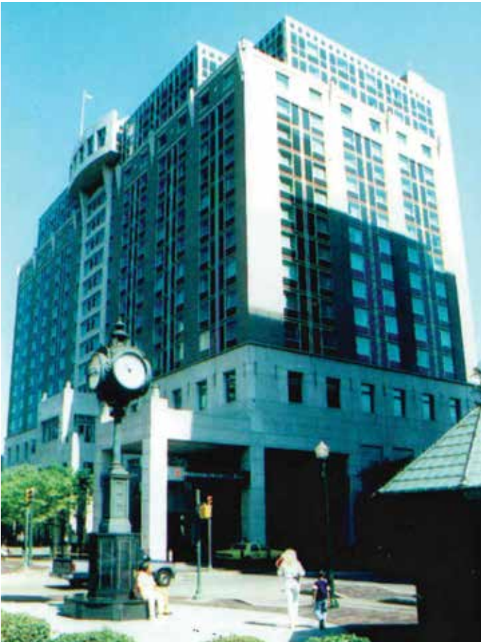
NEWLY CONSTRUCTED HILTON HOTEL AT MARKET SQUARE - 1990
