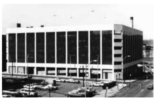
CONSTRUCTION OF 5TH STREET GARAGE - 1978-1979
